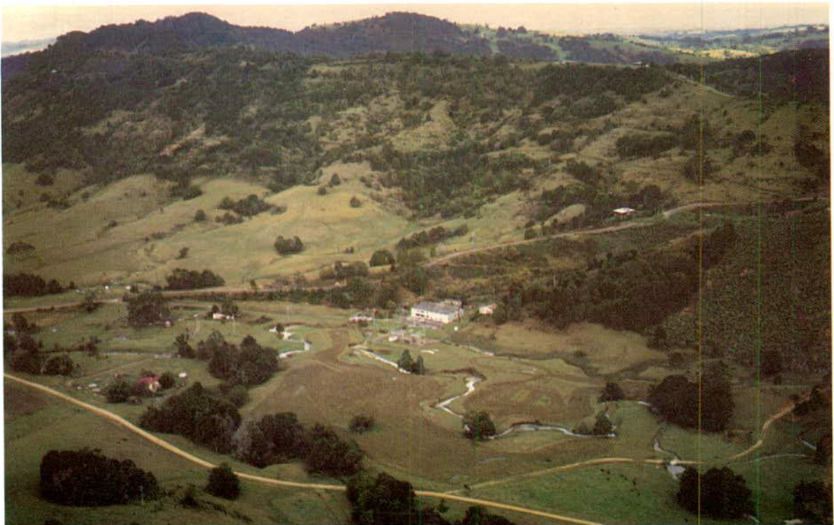
PLATE B.4: Looking south east towards the Mullumbimby Power Station and the coastal escarpment. The line terminates near the Power Station and runs up the escarpment near the middle of the photograph.
